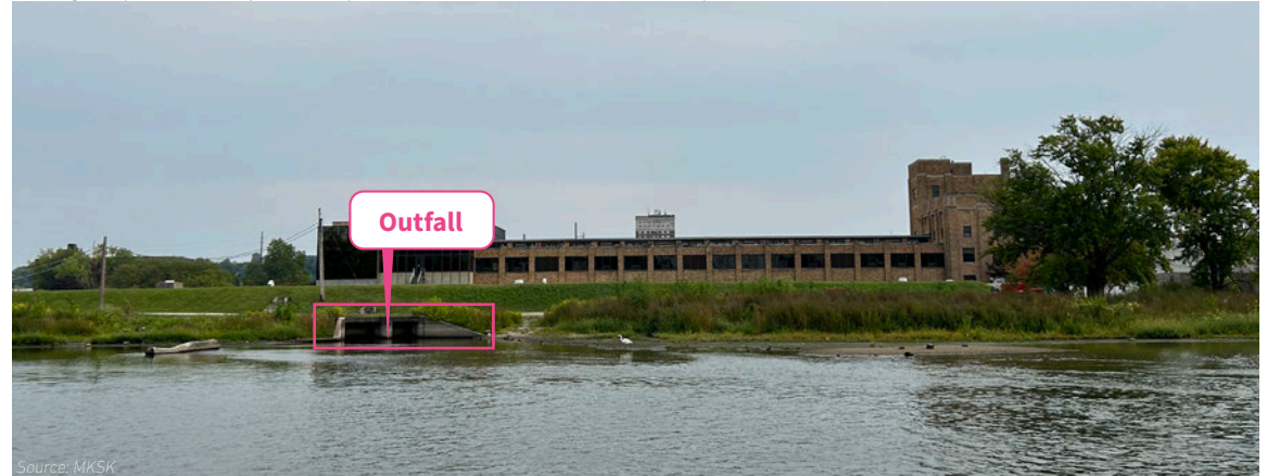
Utility Structures where 20th Street meets the River
